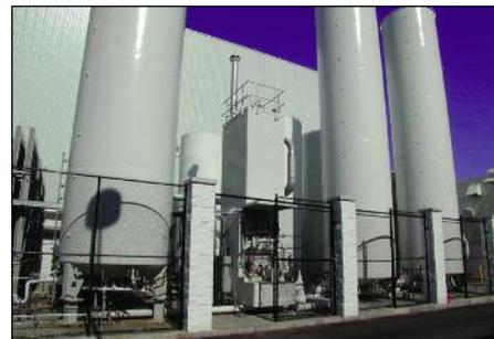
Argon recycling system based on liquefaction
