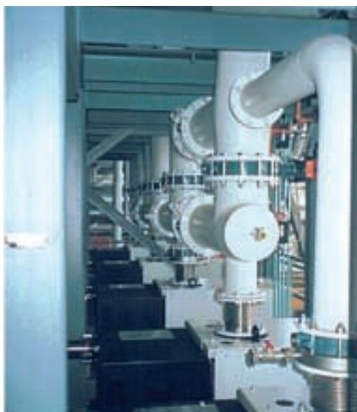
**Vacuum pump system of a continuous freeze-drying plant**
